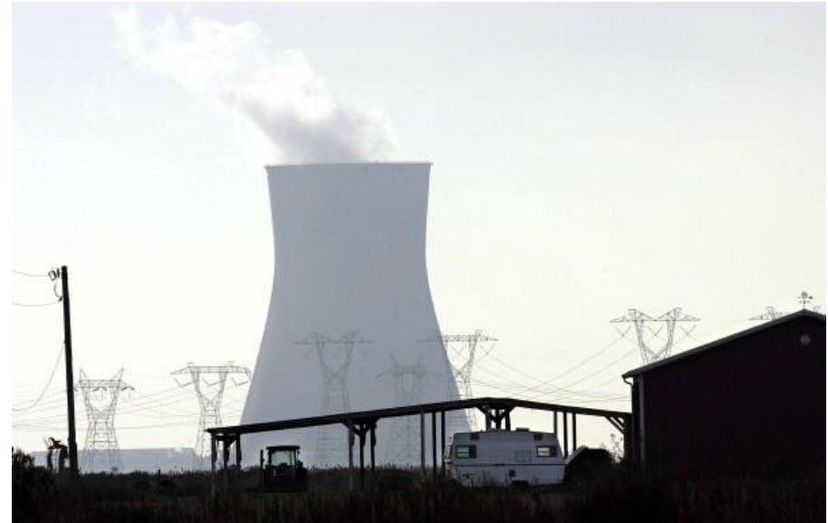
PSEG nuclear plant in New Jersey
